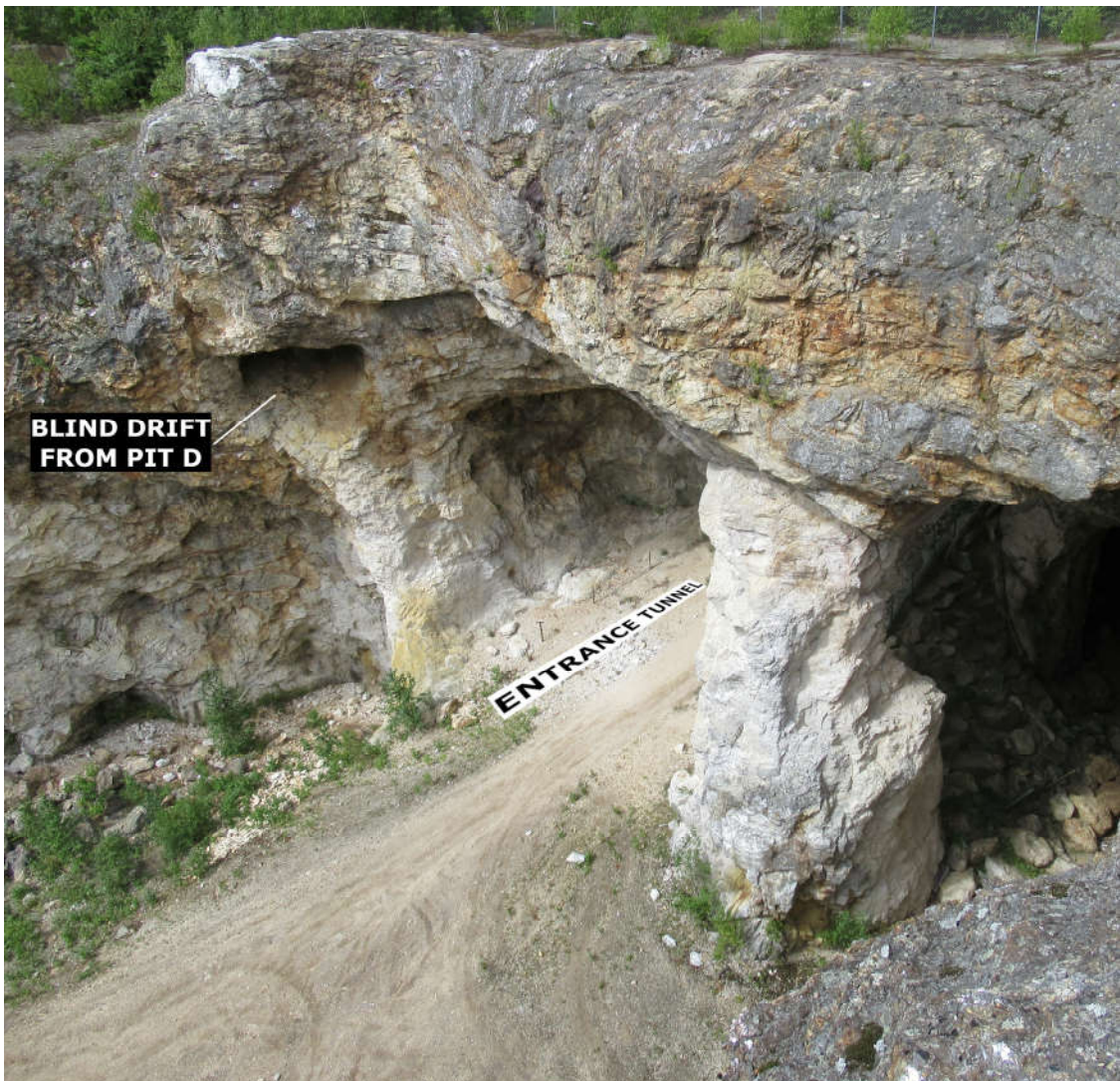
Figure 27. Blind drift, formerly in the wall of Pit D of Cameron in 1944 [Figure 1: 10; Figures 12 & 13], now above the entrance tunnel to the parking lot. Viewed from above. Photo by the author, 2020.
