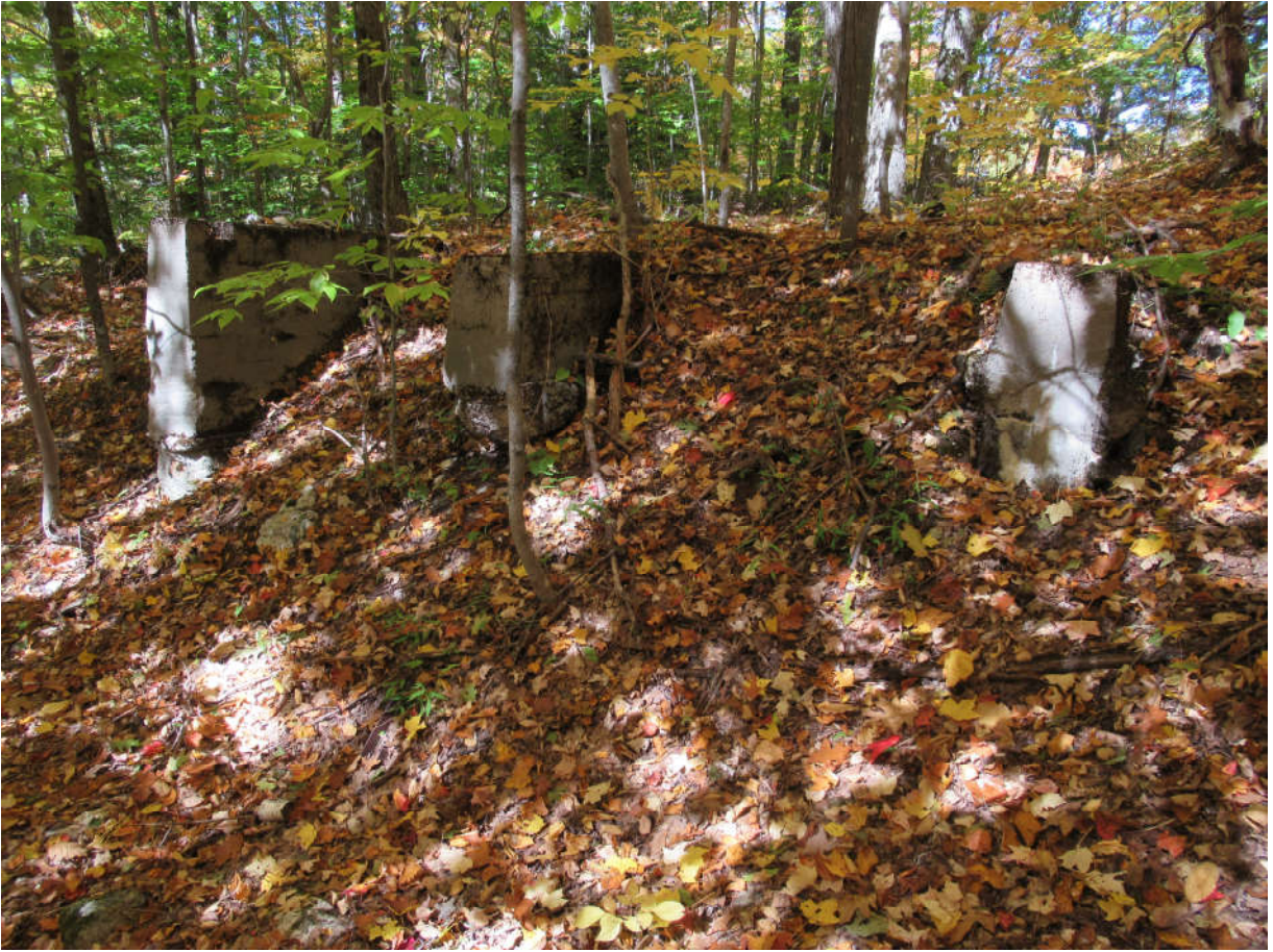
Figure 26. Concrete structures outside the northwest corner of the open pit near the area labeled “Mill” in Figure 10. Photo by the author, 2022.
